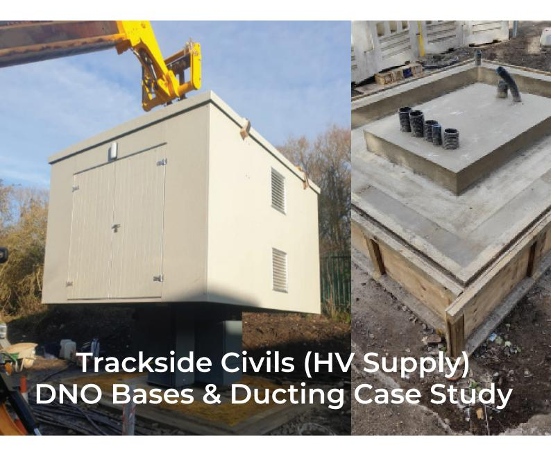
H&A Rail Ltd secured the winning bid to install new RC concrete bases, ducting, NEW TRAIN EV CHARGING POINTS, and STAKKA boxes.
