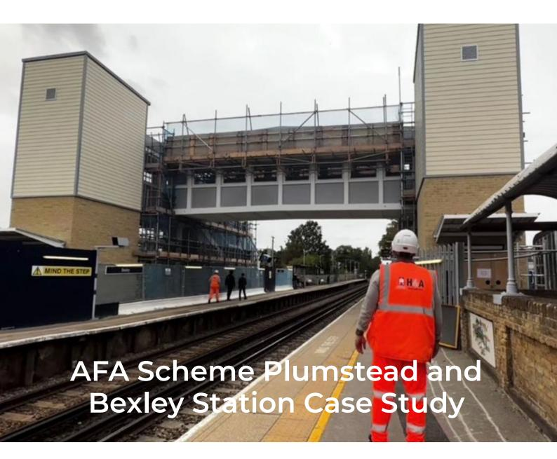
H&A Rail's specialist Brickwork team completed an AFA Scheme, building lift shafts at Plumstead and Bexley stations.
